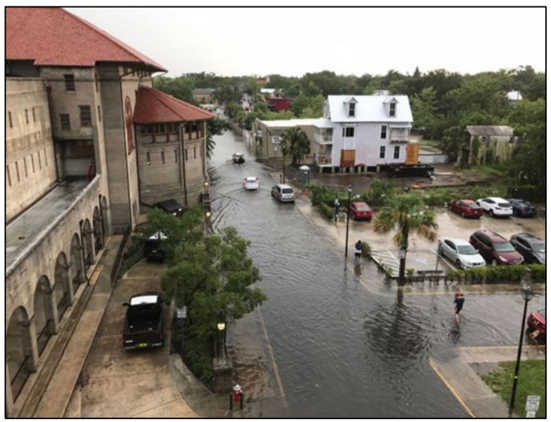
Figure 6. Flooding outside City Hall during Tropical Storm Nicole (USACE, 2023).
