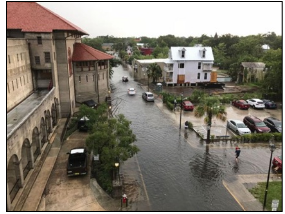
Figure 20. Flooding at S2 during Tropical Storm Nicole (USACE, 2023).
