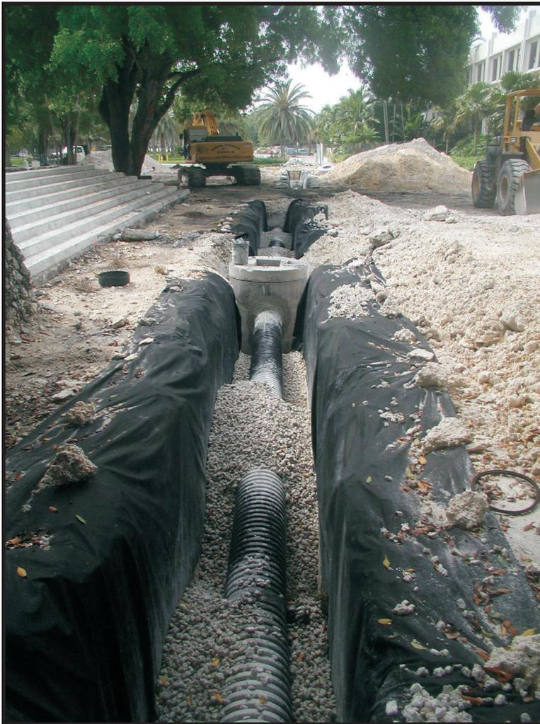
**Figure 1.** Exfiltration trench under construction.
