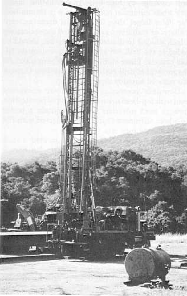
Figure 5-49.—Top-head drive drill with head in mast for drilling. P801-D-81043.
