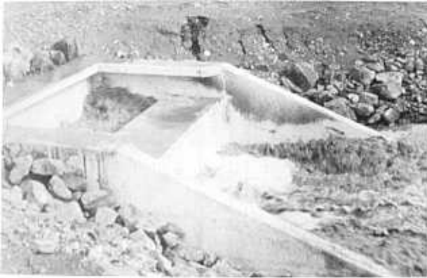
Figure 10-15.—Impact-type stilling basin in operation. 288-D-2905.
