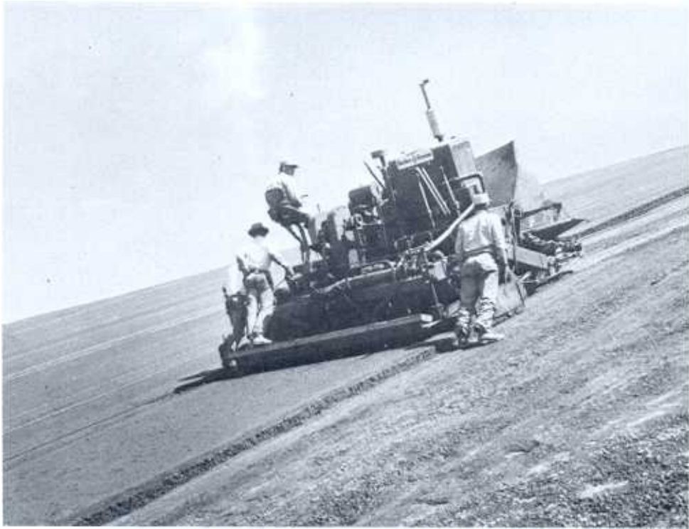
Figure 7-17.—Placing asphaltic concrete on the face of Montgomery Dam, Colorado. CH-520-81.
