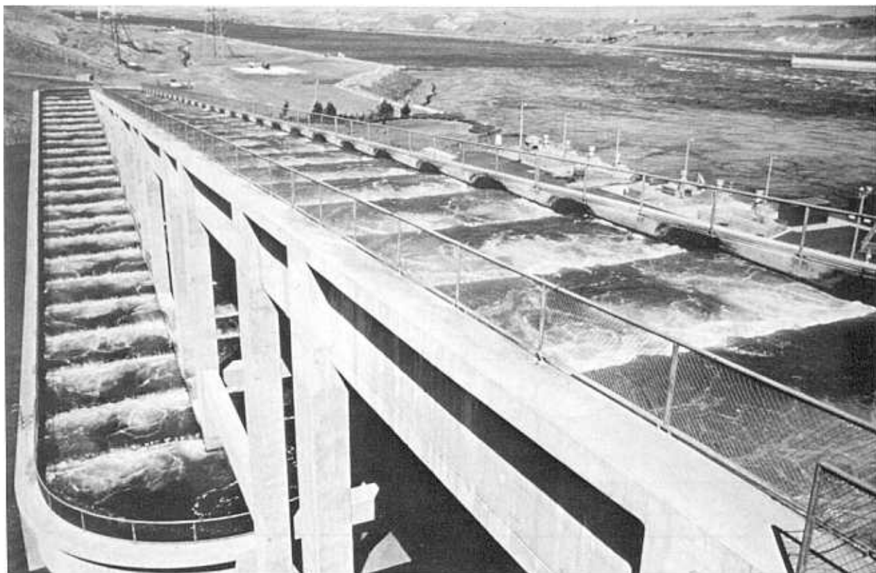
Figure 2-4.—Alaska steep pass fishway, fish ladder. Ice Harbor Dam, Alaska. P801-D-81028
