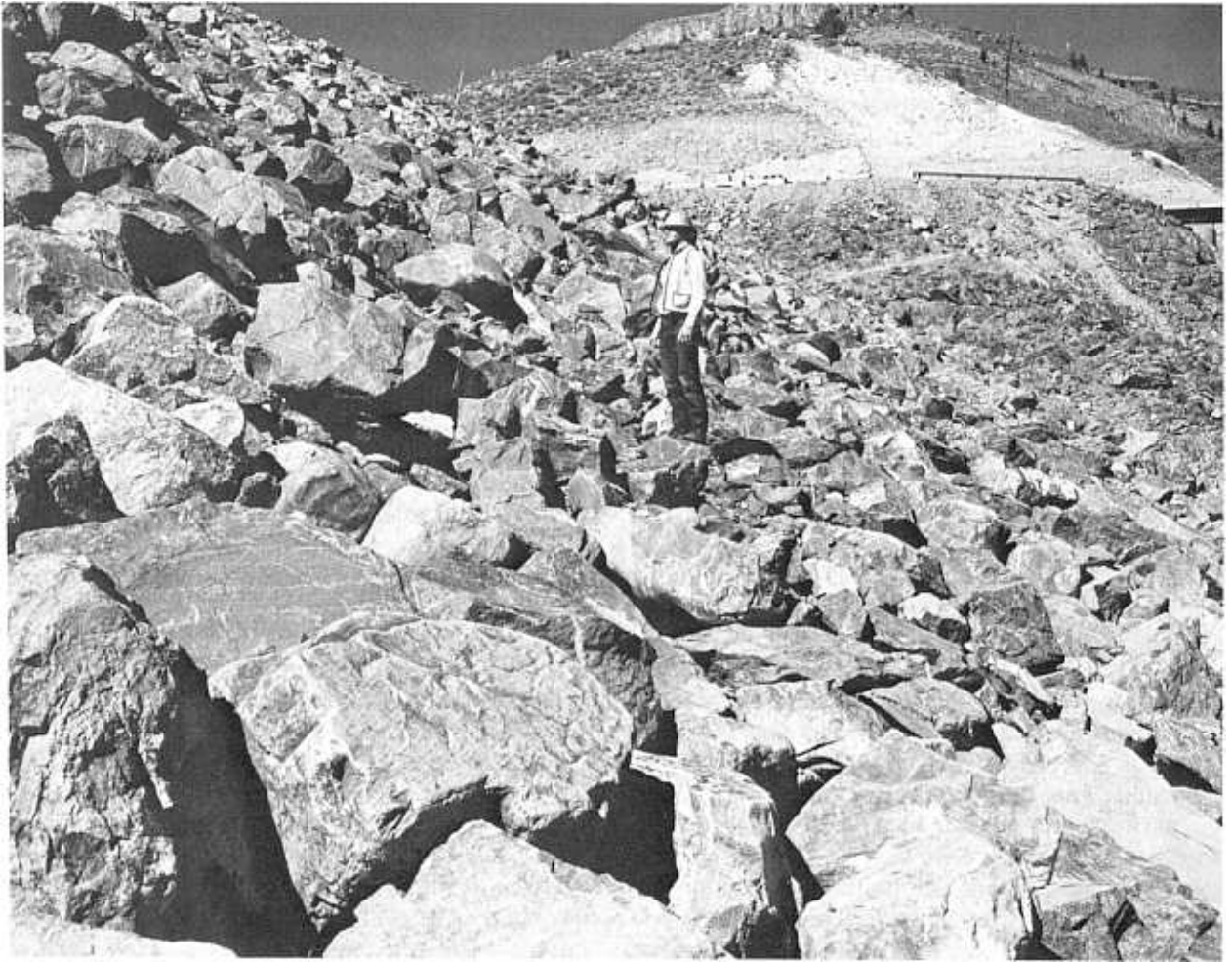
Figure 6-50.—Completed riprap slope protection on upstream face of Blue Mesa Dam, Colorado. P662A-427-10496NA.
