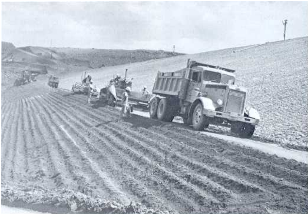
Figure 6-55.—Placement of soil-cement slope protection. Starvation Dam, Utah. P66-418-3549.
