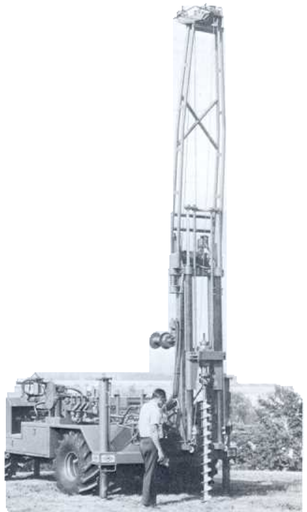
Figure 5-45.—Continuous-flight auger mounted on an all-terrain carrier. D-1635-11.
