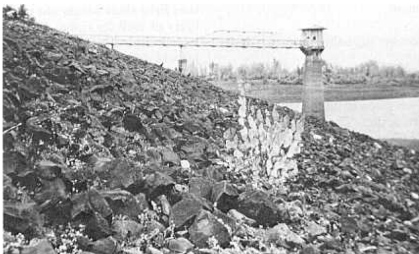
Figure 6-46.—Riprap on upstream slope of an earthfill dam. Dam is in excellent condition after 50 years of service. The structure is Cold Springs Dam, which forms an offstream reservoir on the Umatilla Project in Oregon. IO-2194.
