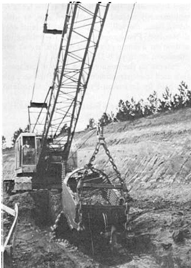
Figure 6-19.—Excavation of a slurry trench. (U.S. Army Corps of Engineers). 288-D-2894.
