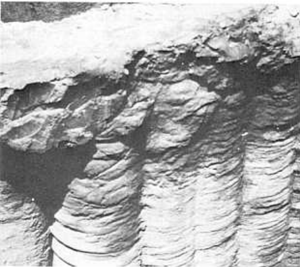
(B) Finished wall. (Intrusion-Prepakt Co.). 288-D-2876.
