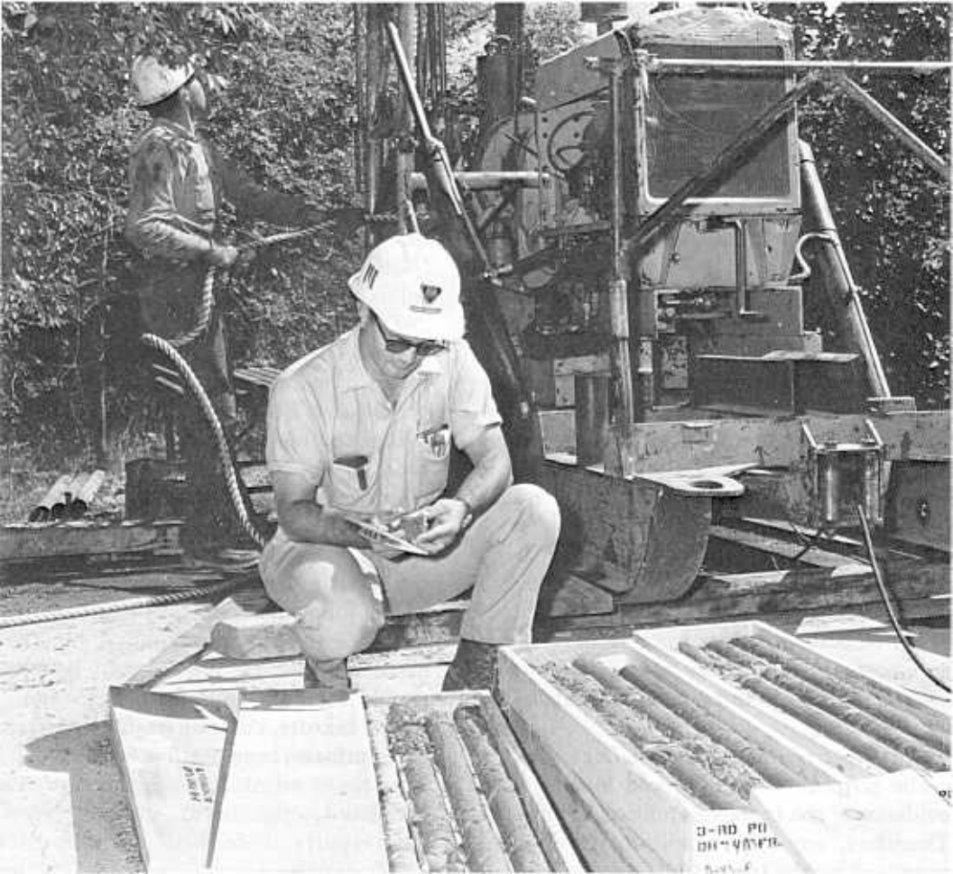
Figure 5-68.—Logging of core obtained from rotary drilling. P1222-142-2198.
