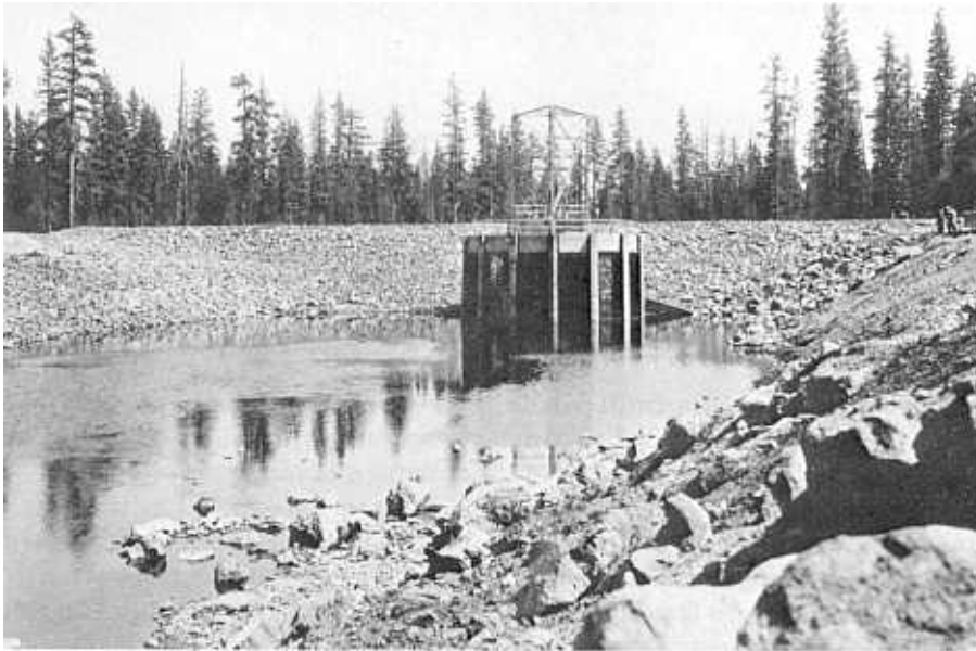
Figure 6-1.—Upstream face of dam and fishscreened inlet structure. Crane Prairie Dam on the Deschutes River in Oregon.
