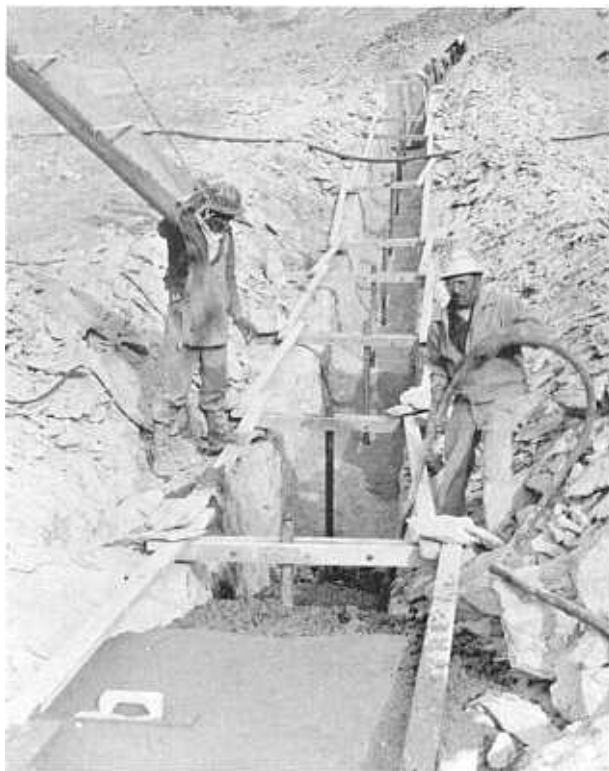
Figure 6-12.—Placing concrete grout cap at Navajo Dam, New Mexico. The 2-inch-diameter grout nipples are fixed at 10-foot intervals. 711-422-250.
