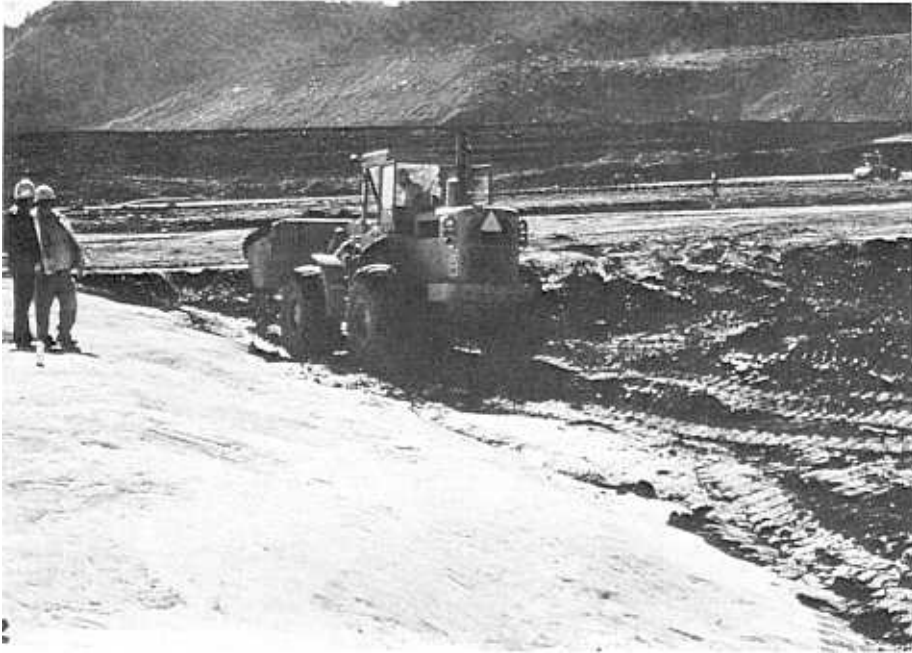
(a) First lift of zone 1 against rock. P801-D-81037.
