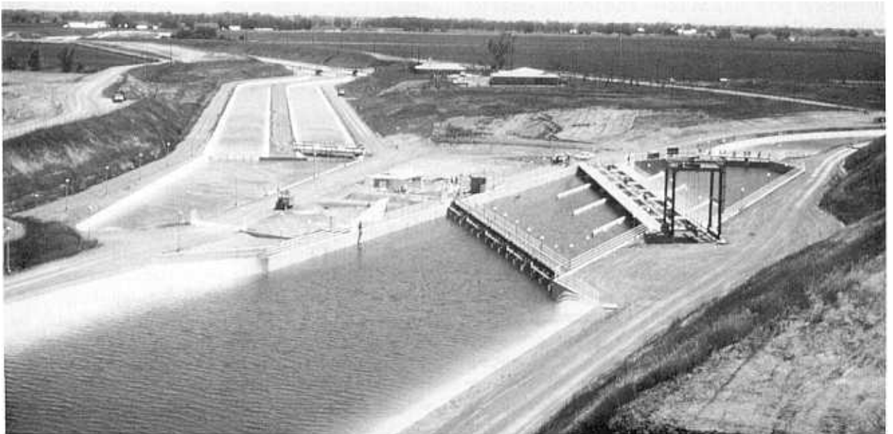
Figure 2-3.—Artificial spawning channels along the Tehama-Colusa Canal. Part of the Central Valley Project, California. P801-D-81027
