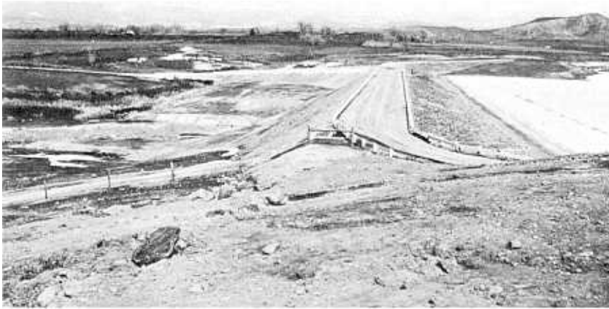
Figure 6-2.—Fruitgrowers Dam, an earthfill storage dam at an offshore location in Colorado.
